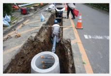
Underground construction to install wastewater piping for factory water discharge (Kyoto Plant)
