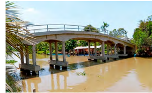
A bridge on the school commuting route
