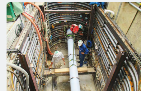
Underground construction to install separate wastewater piping (Kyoto Plant)
