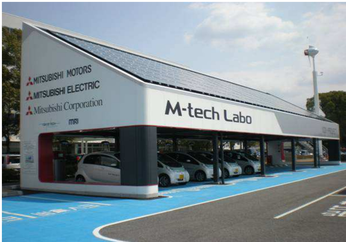
“M-tech Labo”, Smart grid experimental plant
