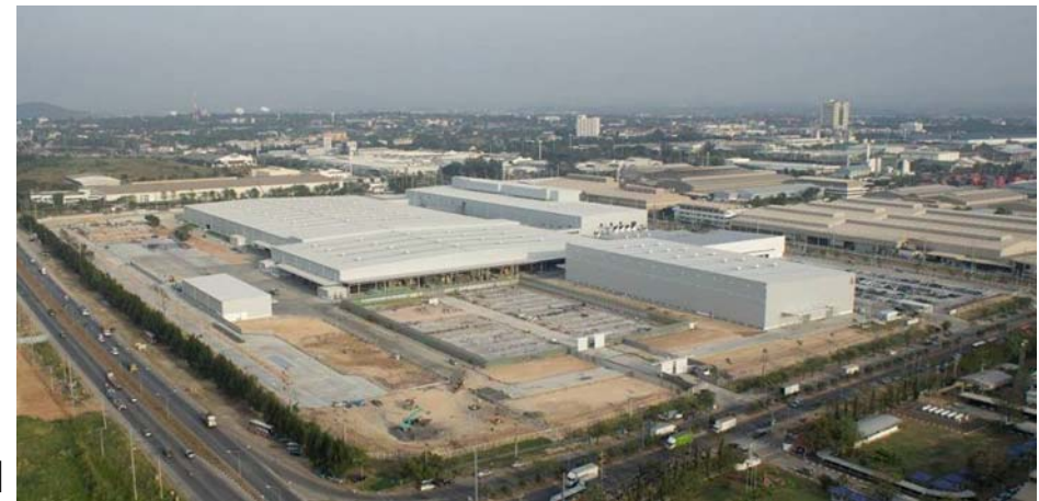
New Third Factory In Thailand (as of December 2011)
