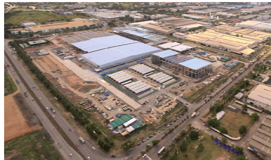
Third Factory (under construction)
