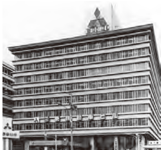
Mitsubishi Motors' head office building (in 1970)
